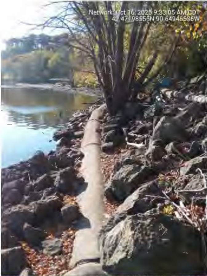
Some exposed sections of the Dubuque Forced Sewer Main. Photos taken 10/16/2020.
